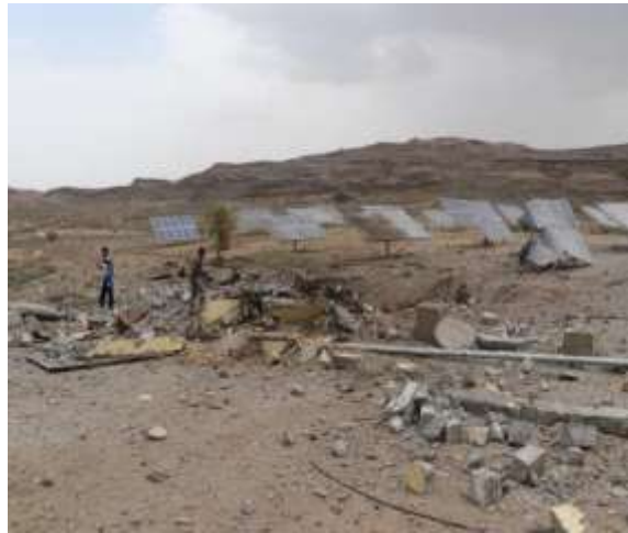
Figure 33.D.3 Site after the attack 81
