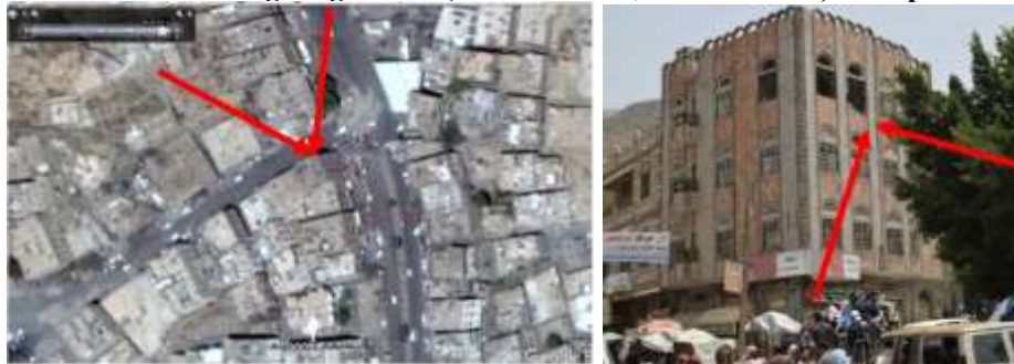
Figure 35.D.1 Location of building targeted at (13°34'9.51"N, 44° 0'0.01"E) with potential direction of attack
